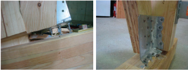
Photo7 Failure condition of J-cy-1_re
